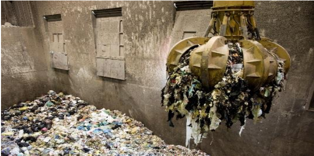
Non recyclable waste plant
